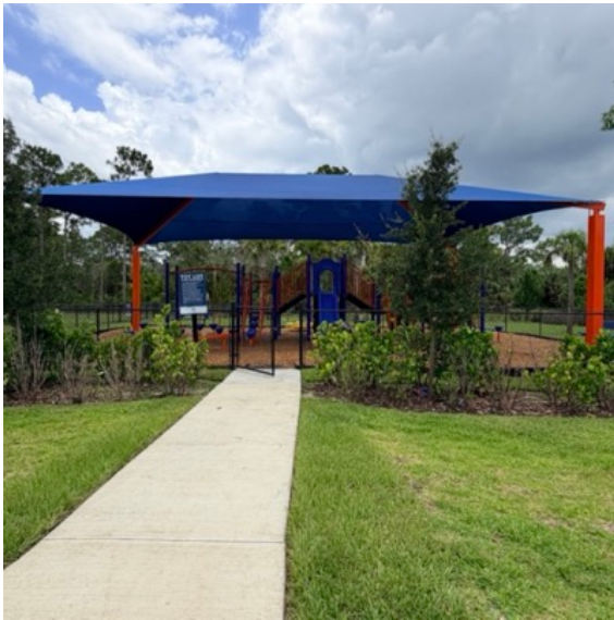
Observed playground with ADA access
